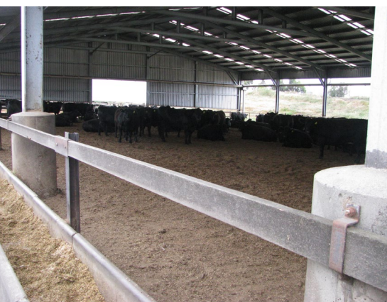
Gable, trussed roof with sheeted end wall
