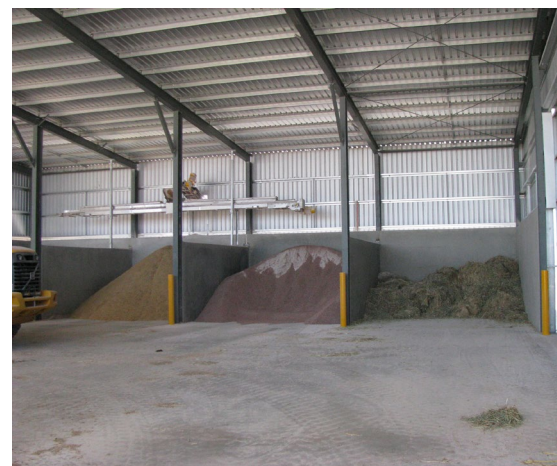
Commodity storage shed with multiple storage bays.
