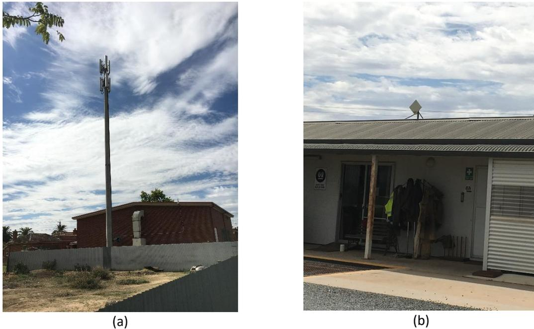
*Figure 3-18. (a) NBN fixed wireless tower in a rural town and (b) fixed wireless antenna (diamond shaped) on a nearby feedlot office (4 km away).*
