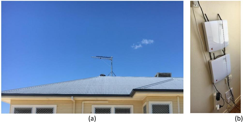
*Figure 3-4. (a) An example of a dual mobile booster located on the roof of a feedlot office, and (b) the internal router boxes used to (internally) link office desktops. Note the mobile link is facilitated by a Yagi antenna. A second Yagi (directly beneath the first) is used for the point-to-point link (Wi-Fi) to an Induction shed*
