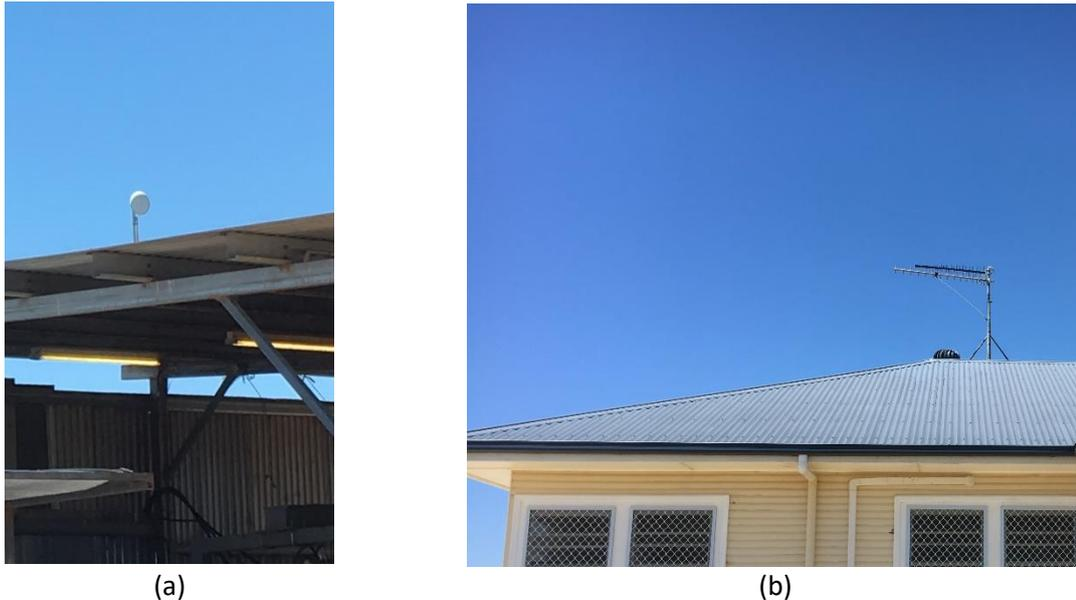
*Figure 2-11. Examples of a point to point link between (a) an induction shed and (b) feedlot office. The induction shed has a parabolic dish and the feedlot office uses a Yagi to facilitate the link.*
